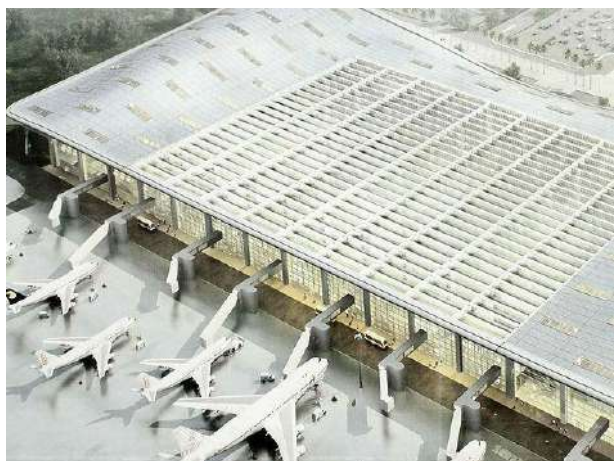
Airside view of upgraded T-1
