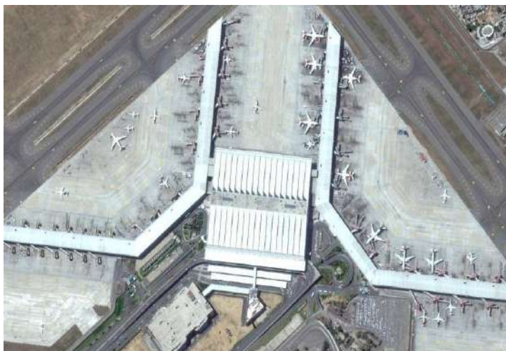
Delhi Airport Terminal-3
